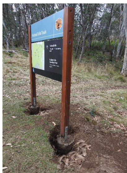
Soil dug away from the base of the signs at Federal Falls Picnic Area. Photo R Stapleton.
